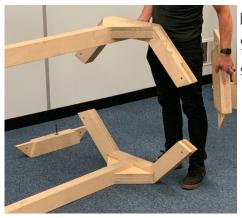
Lift the Upright and slot in the Base Struts. The portals base is octagon shaped.
