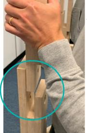
The staggered design at the fixing point will guide and support as you assemble.
